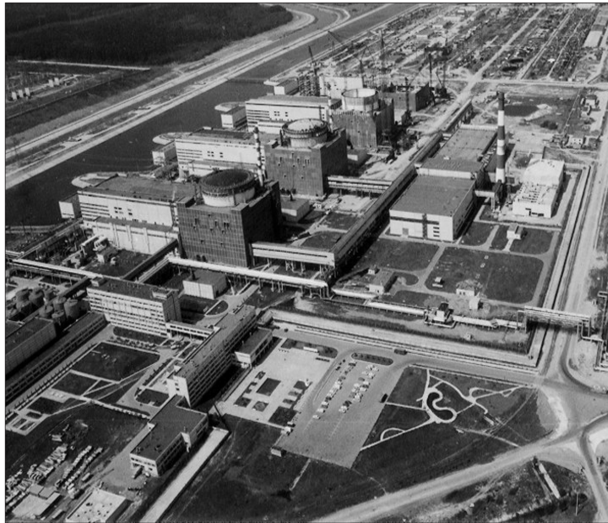
The Bushehr nuclear power facility in Iran
